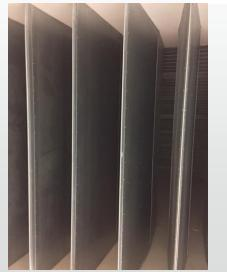
3 sections of ducted silencers to minimise transmitted noise along the wind tunnel
